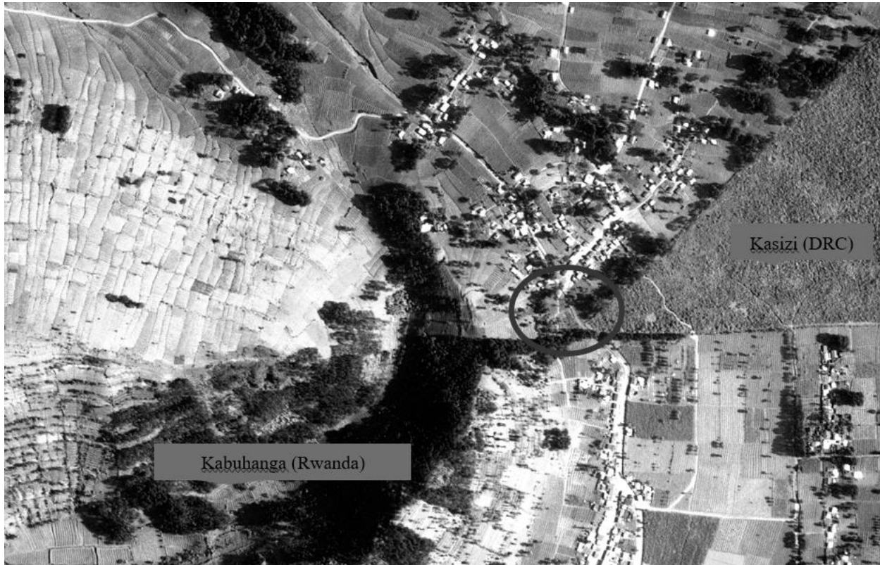
Planet™ satellite image on 05 October 2024, annotated by the Group of Experts
