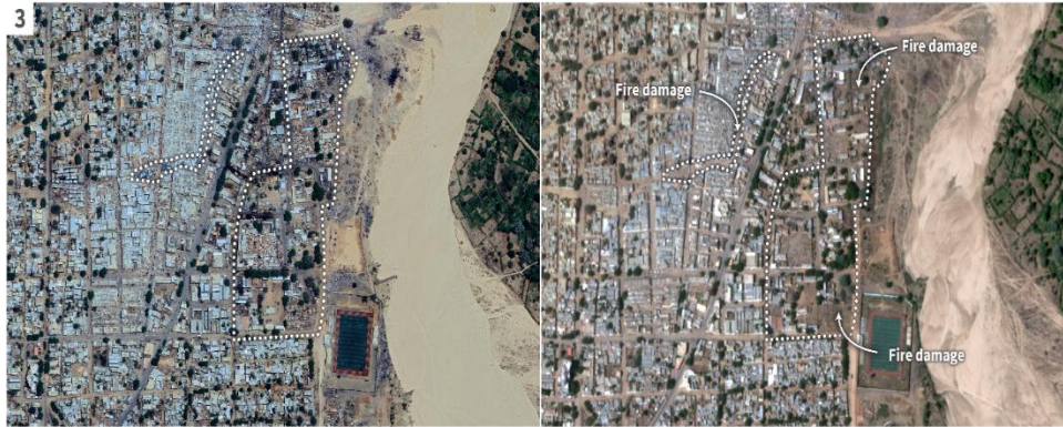
Satellite imagery of fire and infrastructure damage in Al Nahda North and Al Zuhur neighbourhoods, east El Geneina. Left image-Obtained 19 April 2023. Right image-Obtained 17 November 2023.
