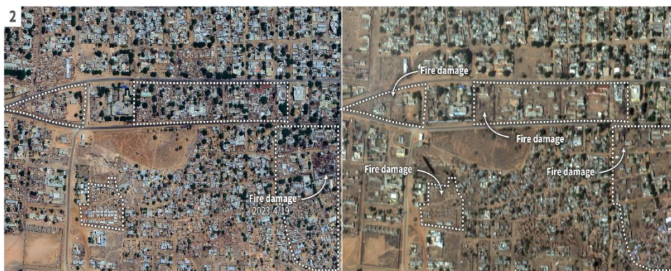
Satellite imagery of fire damage at IDP gathering locations and infrastructure damage in Majlis and Al Tadamon neighbourhoods, El Geneina. Left image-Obtained 19 April 2023. Right image-Obtained 17 November 2023.
