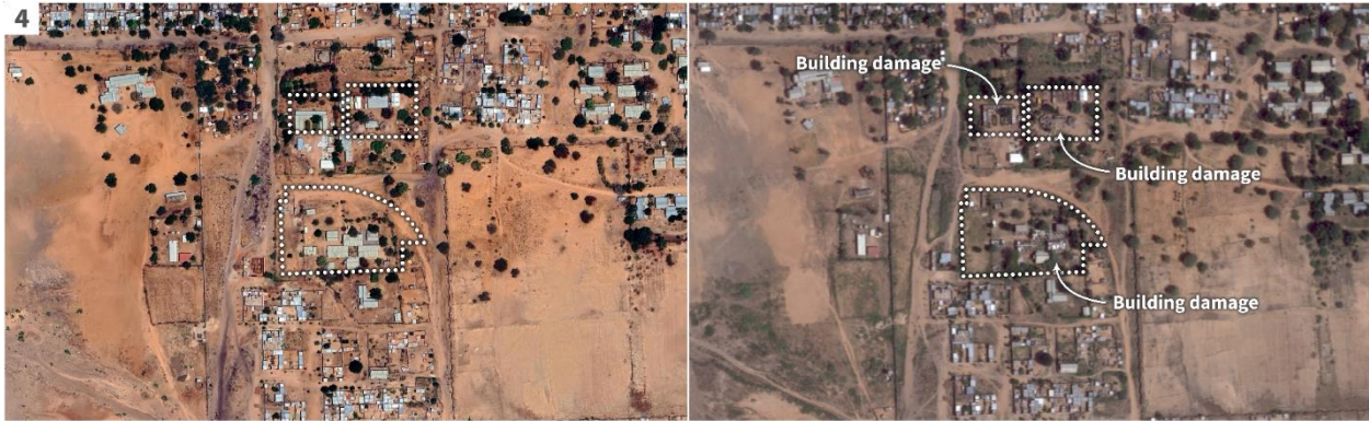
Satellite imagery showing damage to government and educational buildings in Karari East neighbourhood, Nyala, southeast from the SAF 16 Infantry Division. Left image-Obtained: 8 Apr 2023. Right image-Obtained 24 October 2023.
