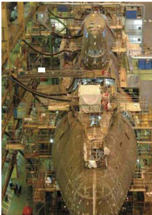
HMS ASTUTE under construction at BAe Systems Submarines, Barrow-in-Furness (picture courtesy of BAe Systems)
